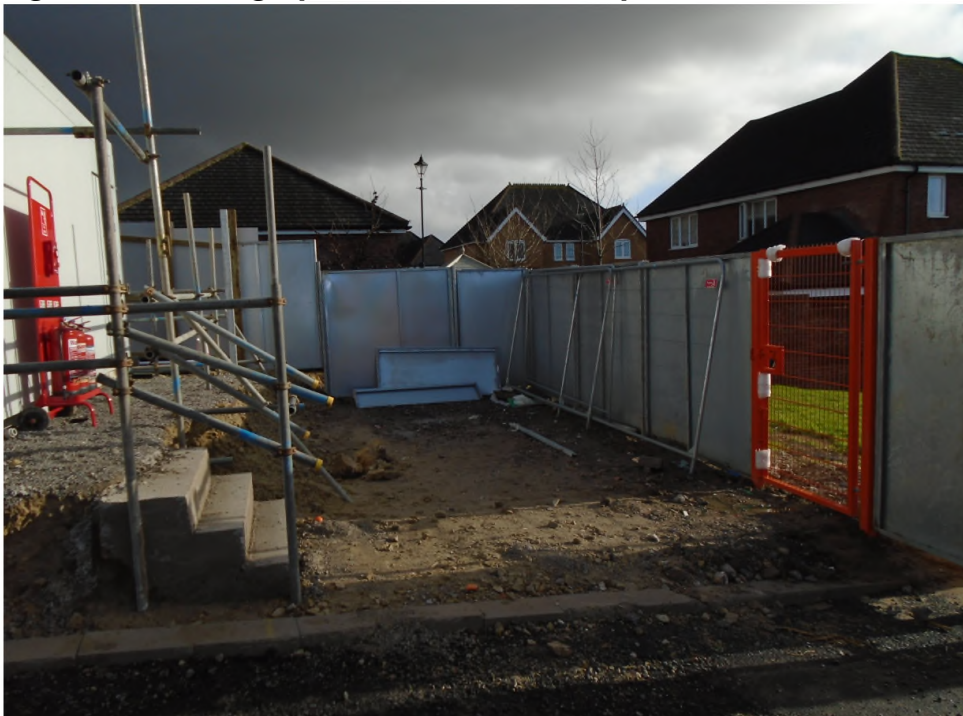
Figure 4 – Photograph of Location of Proposed Sales Suite Building
